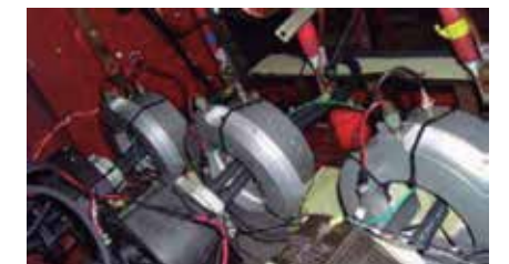
Fig.6 HSCT Sensor (high sensitivity current transformer)
